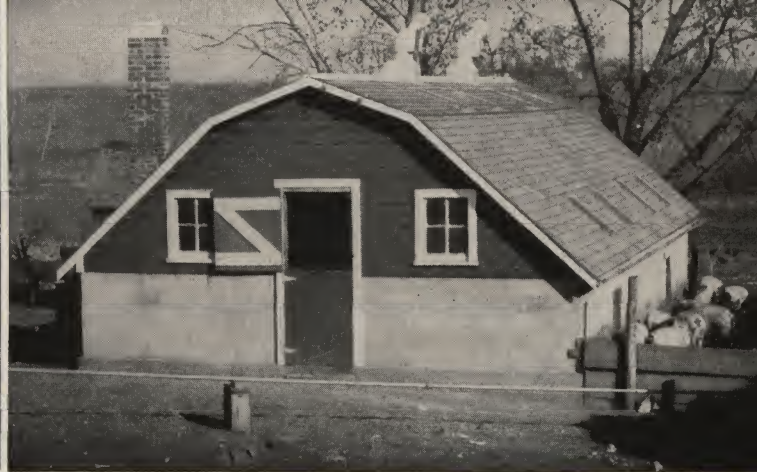
Good examples of the modern gable roof and gambrel roof hog houses. Houses like these in the northern half of the United States should have insulated ceilings about 7 ft. 6 in. above the floor to provide a warm house for early spring farrowings.
